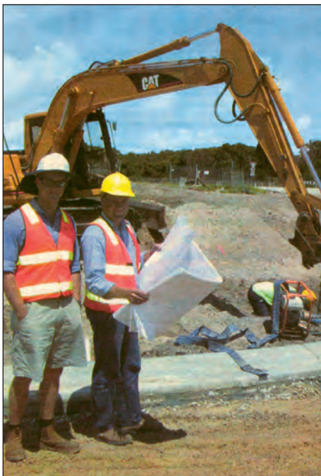
Hutchies is the Design and Construction Manager for the Casuarina Beach project, with Site Foreman, Jeff Miller (right) and building cadet, Rob Archibald, pictured on site.
