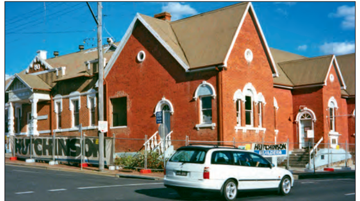
Hutchies' experience of working on heritage listed buildings helped win the contract for restoration of the School of Arts in Tenterfield, New South Wales.
