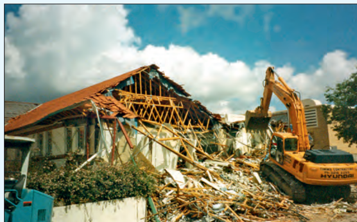
Demolition makes way for new Coles store in Racecourse Road, Ascot.
